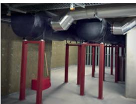
A **double exhaust silencer system** was incorporated, which maintains the backpressure of the equipment and ensures minimal noise. To minimise noise pollution, the sealed room in which the generator sets are located was completely soundproofed, including motorised grilles in the air vents to cool the room, and bushings, which absorb vibrations from the generator sets and the structure supporting the silencers.
