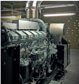
Two HTW1550 T5 generator sets with Mitsubishi engines were supplied. They are **emissions-compliant models** that comply with French law No 2910, which requires engines, between 2 and 20 thermal MW, to meet NOx and HCH emissions limits.
